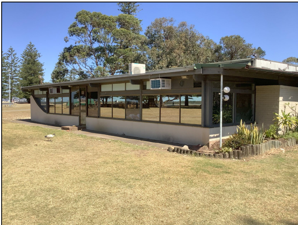
Figure 3-5: View of the existing Dolls Point Café, facing southwest, showing the c. 1980s extension, including tinted, aluminium framed windows and flat roof.
