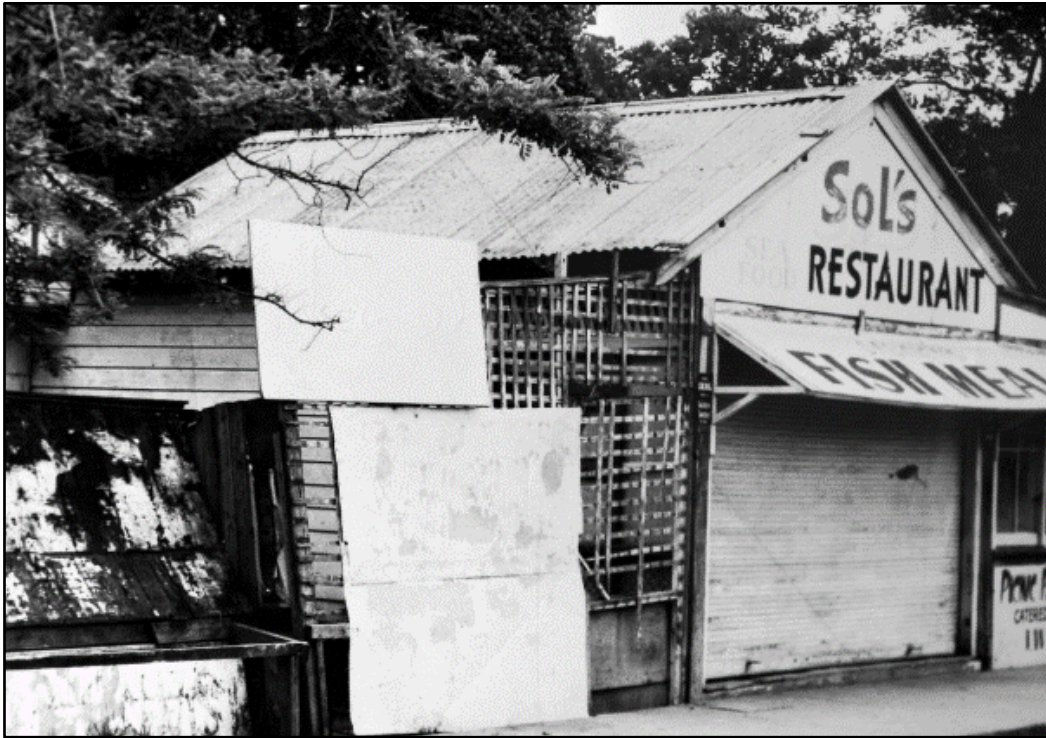
Figure 2-6. Sol's Restaurant closed and boarded up in preparation for demolition, 1961 (Source: Bayside Library Services).
