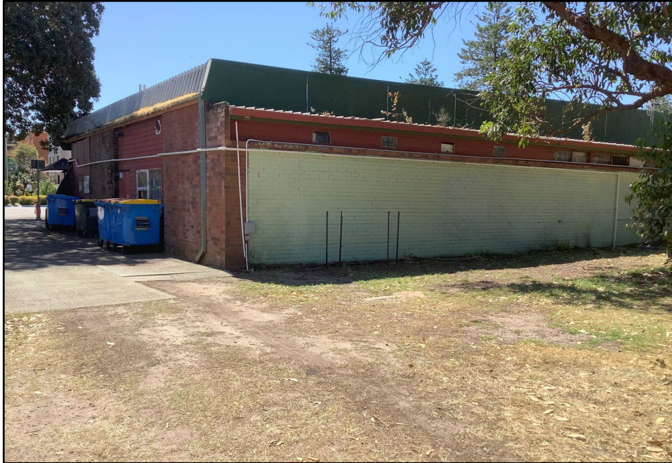
Figure 3-6: Northern facing view of the existing Dolls Point Café, showing the rear of the building. Including brick masonry walls and corrugated metal roof.
