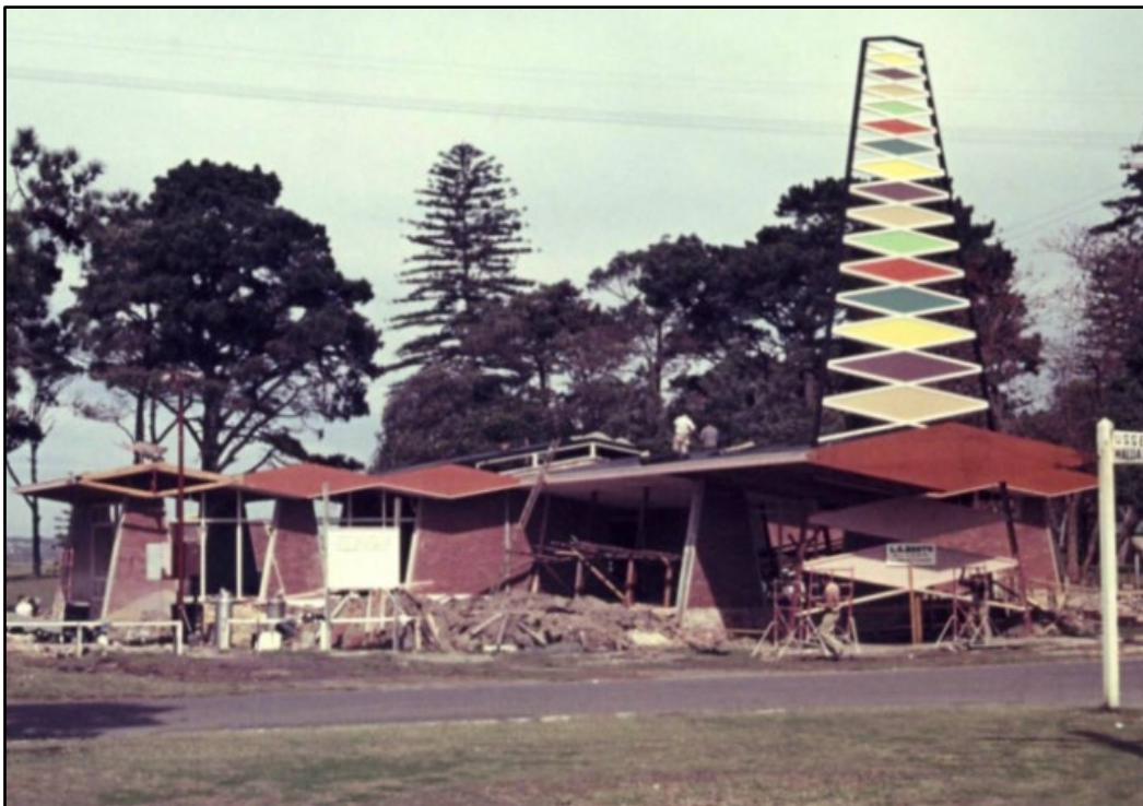
Figure 2-7. The Dolls Point Kiosk, including the tower with geometric design, under construction during 1961 (Source: Bayside Library Services).
